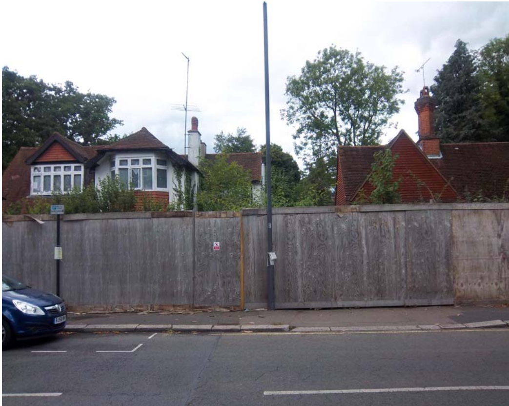
View of 16 and 14 and their position close to the front of Gordon Avenue
